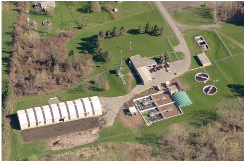
Town of Ontario WWTP with Composting Facility
